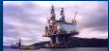
Hibernia platform during tow out
